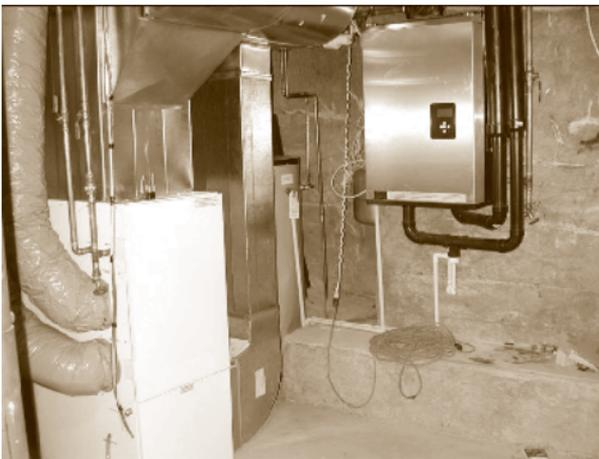
Some early “combination” systems used conventional, natural draft water heaters and a fan coil to supply space heating. These units have low efficiency that makes them unsuitable alternatives to current code-compliant systems.
